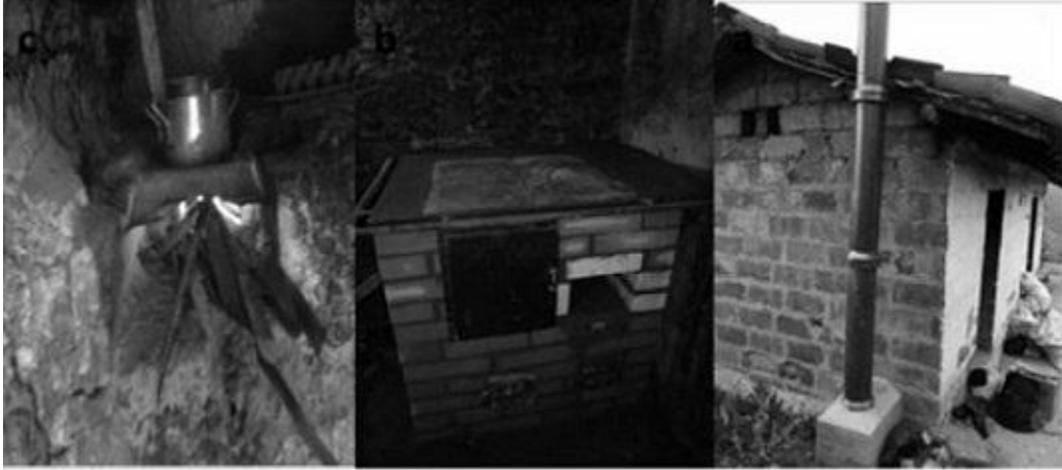
Figura 10.1. Stove made of brick with a chimney pipe.
